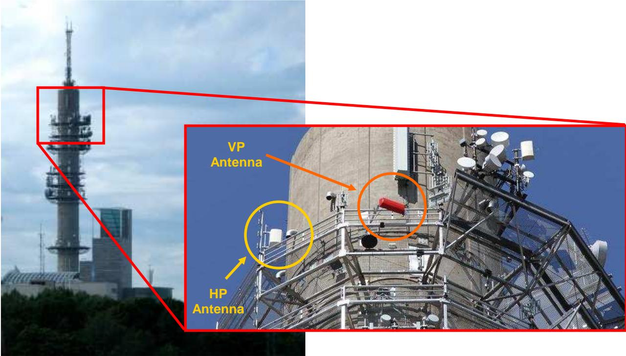
**Figure 3: YLE Transmission Tower at Pasila & the transmitting antennas**
