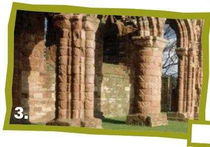
**3. Big pillars inside** – to strengthen the building and hold the heavy roof up.
