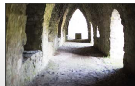
These 'cathedral' like Lime Kilns show the wealth of the area during the industrial boom here.
