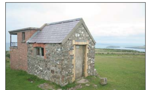
This ruined hut used to be a coastguard look-out
