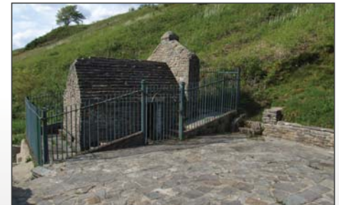
This tiny building holds a well that possibly dates to Celtic times
