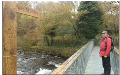
Footbridge into Parc Meurig over the Afon Ogwen
